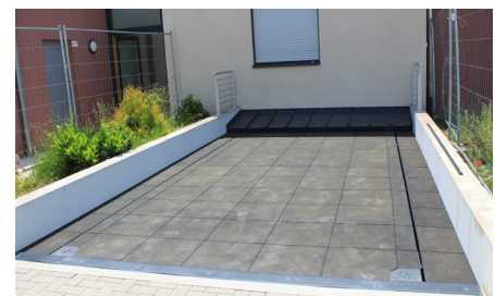
Rubber covering in stone structure (3 cm thick)
