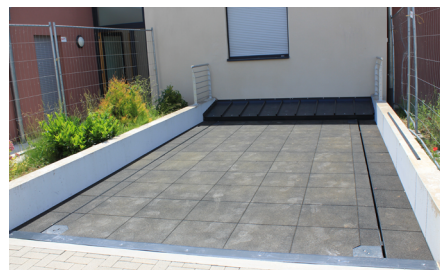
Rubber covering in stone structure (3 cm thick)
