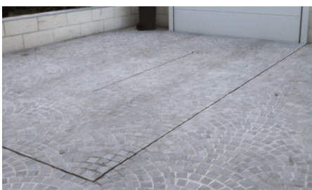
Synthetic stone covering (3 cm thick)
